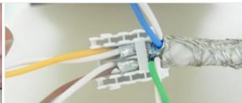
Strip 40mm of sheath from cable using stripper then roll back Separate the four pairs and remove the foil wrap from around Insert front wires under the cross piece with the rear wires sitting at the back.
